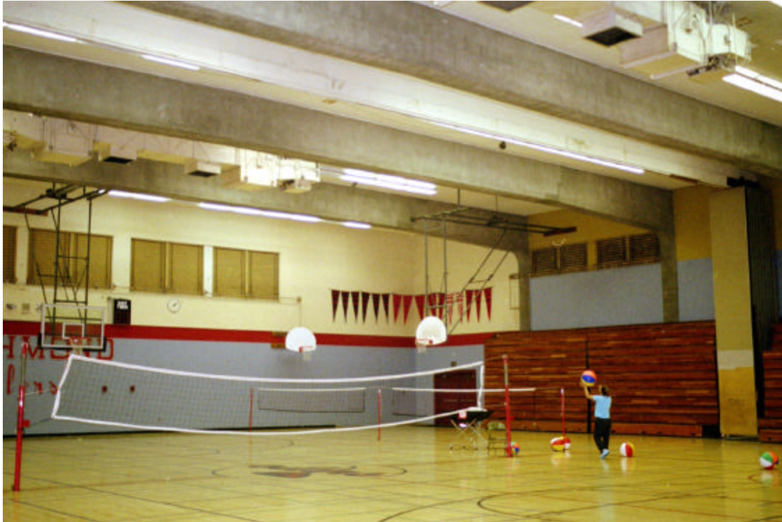
Figure 18: Gymnasium Building (Unit E), interior southeast corner
