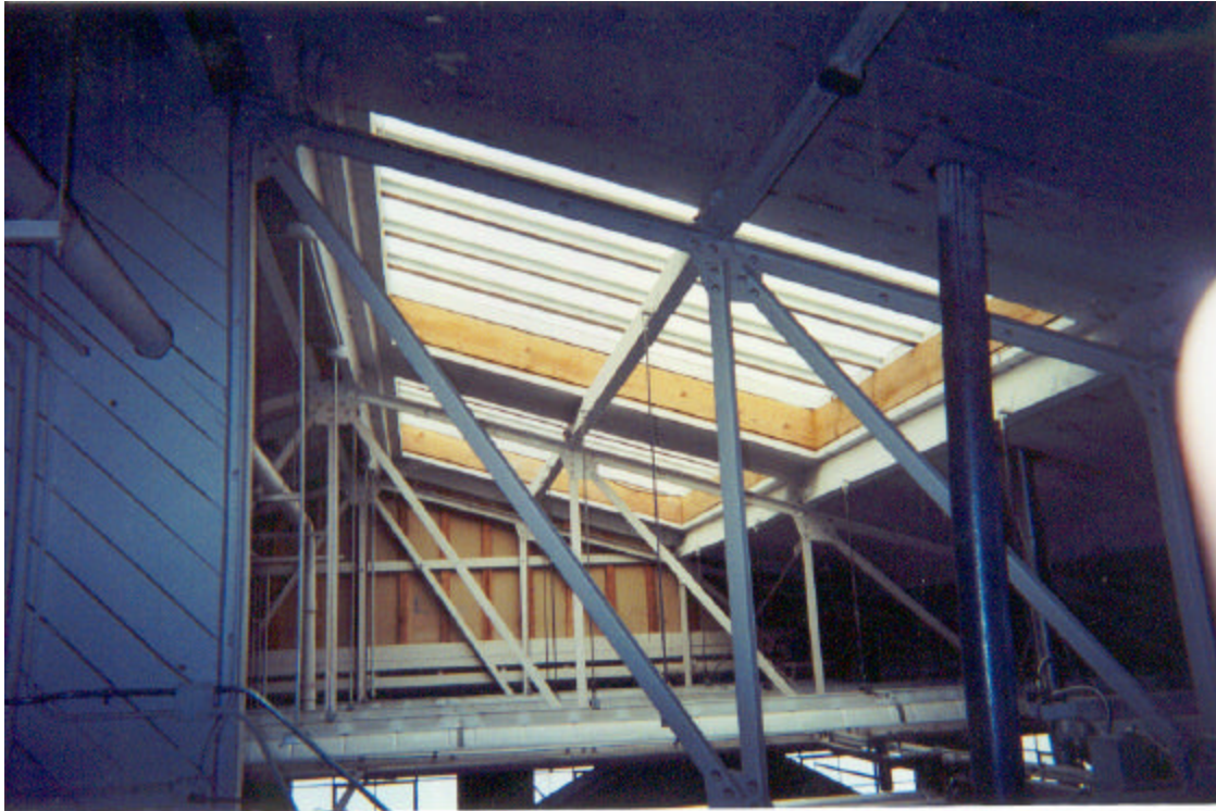
Figure 24: Shop Building (Unit A), interior at roof framing
