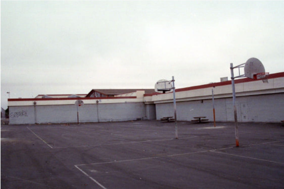
Figure 5: Classroom Building (Unit D), exterior east wall
