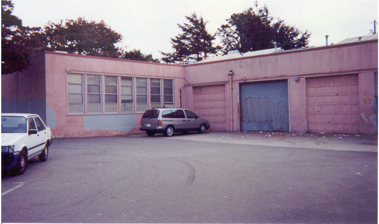
Figure 22: Shop Building (Unit A), exterior north and west walls
