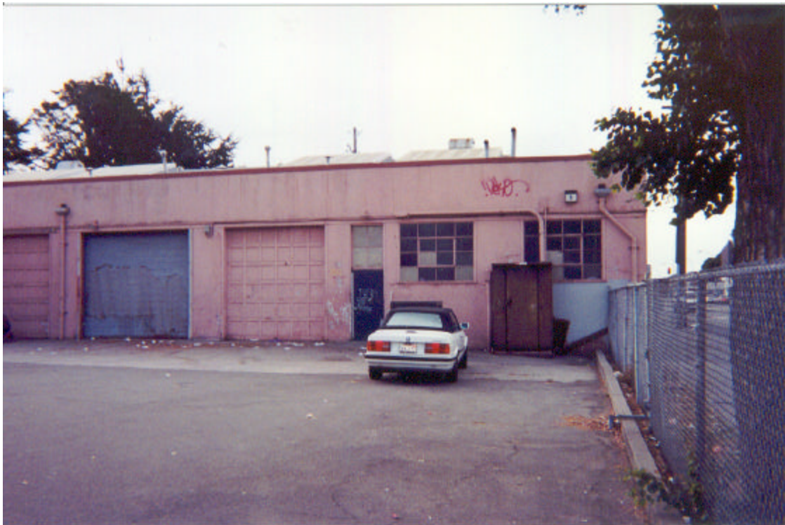
Figure 23: Shop Building (Unit A), exterior north wall
