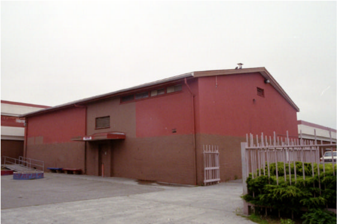
Figure 21: Music Building (Unit F), exterior northwest corner
