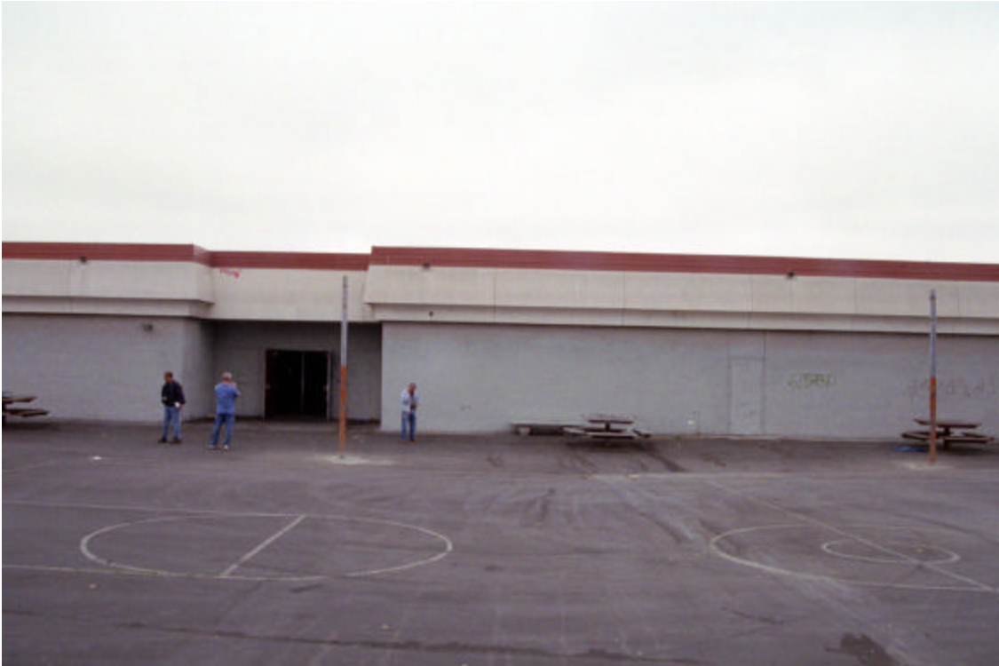
Figure 4: Classroom Building (Unit D), exterior east wall
