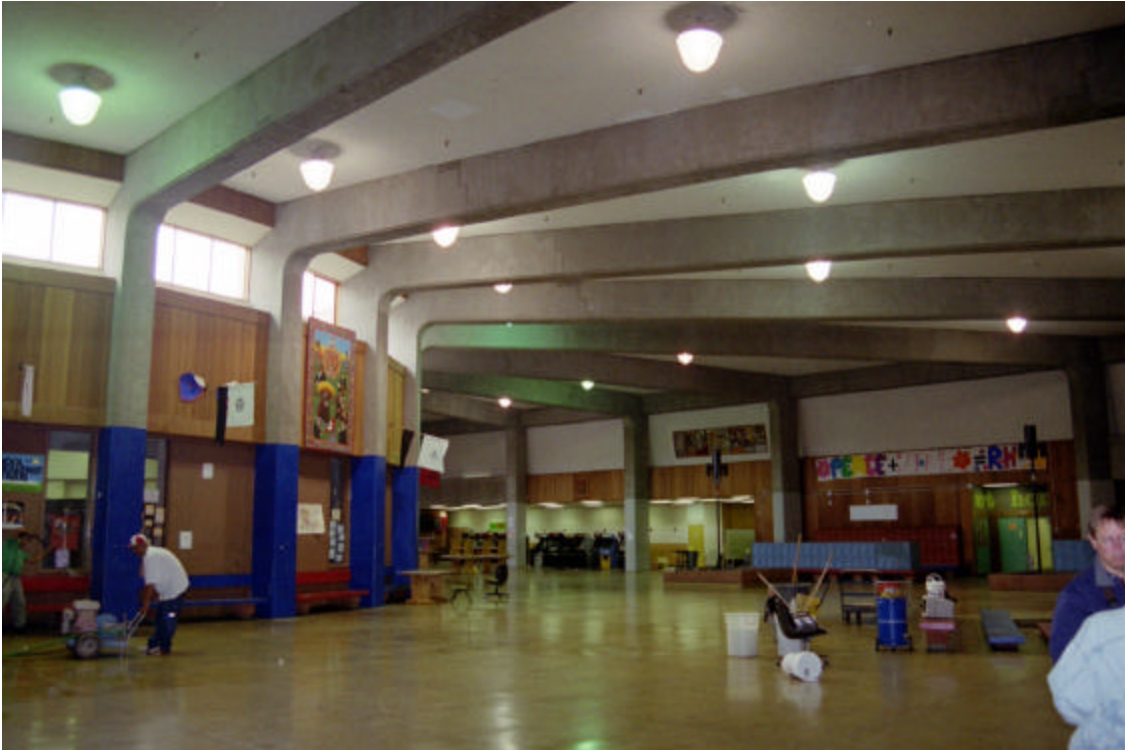
Figure 10: Common Area (Unit D), interior facing clerestory windows
