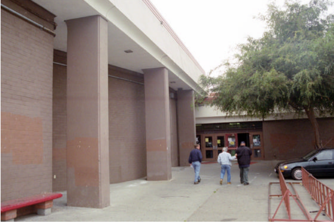
Figure 3: Theatre Building (Unit D), exterior east wall
