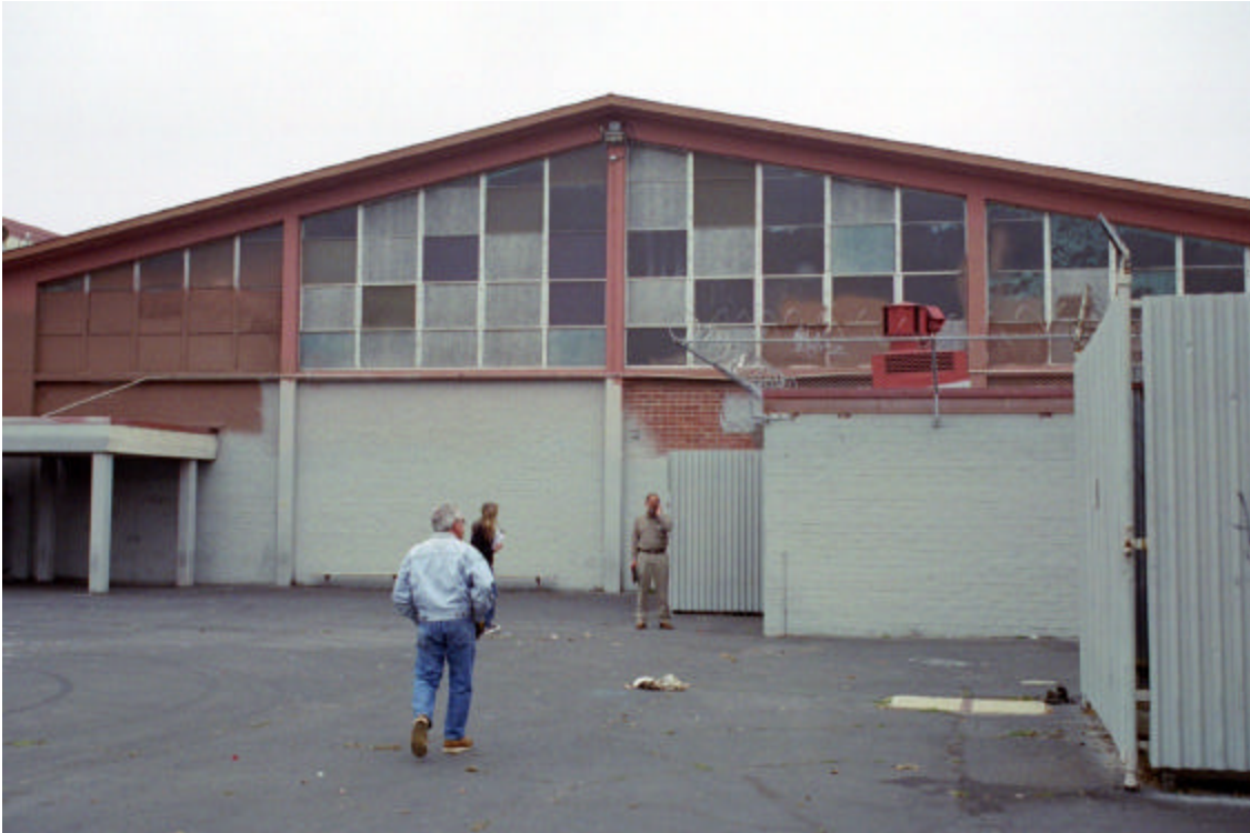
Figure 12: Old Gymnasium Building (Unit B), exterior east wall
