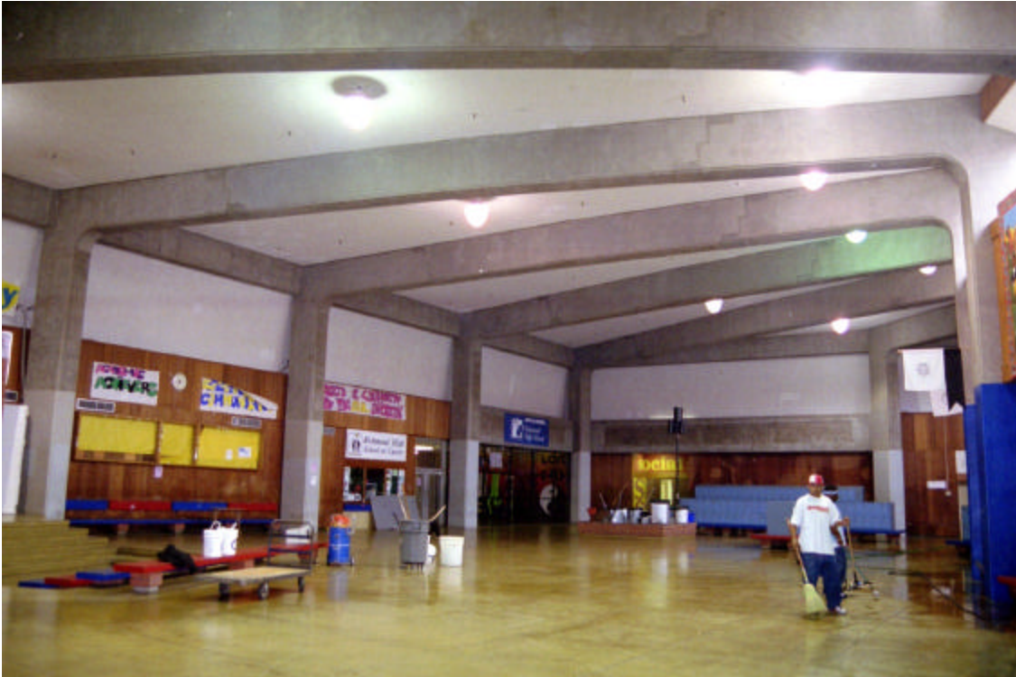
Figure 6: Common Area (Unit D), interior southwest corner
