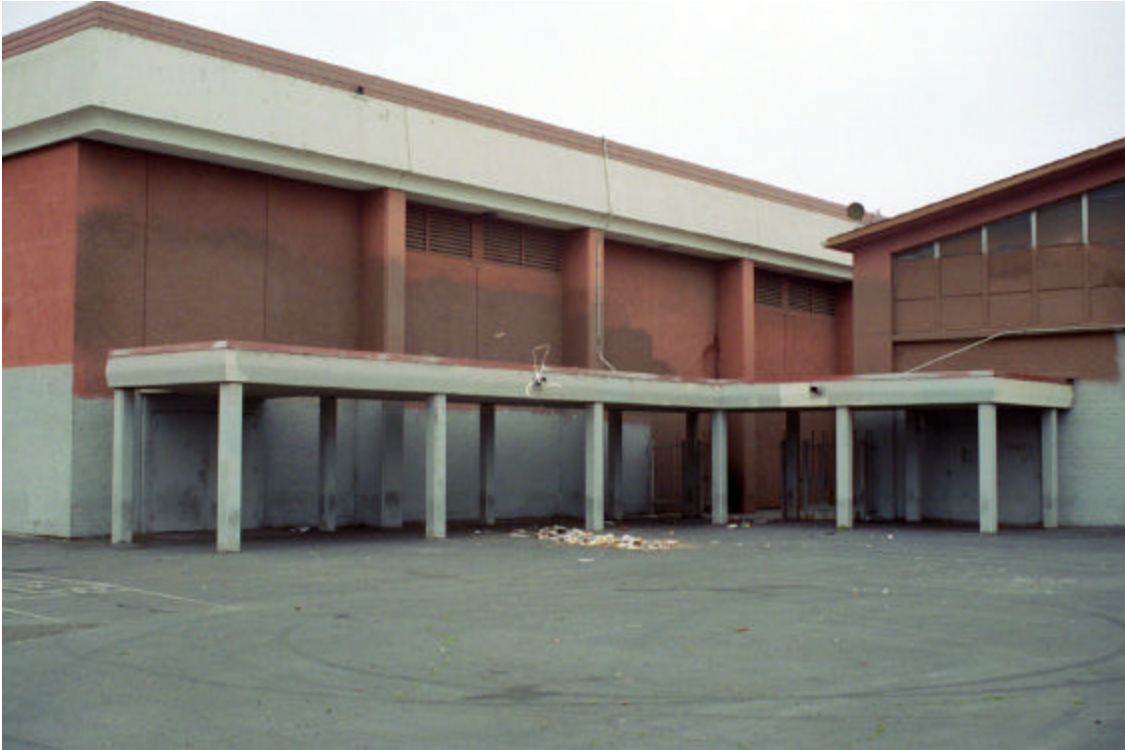
Figure 17: Gymnasium Building (Unit E), exterior north wall
