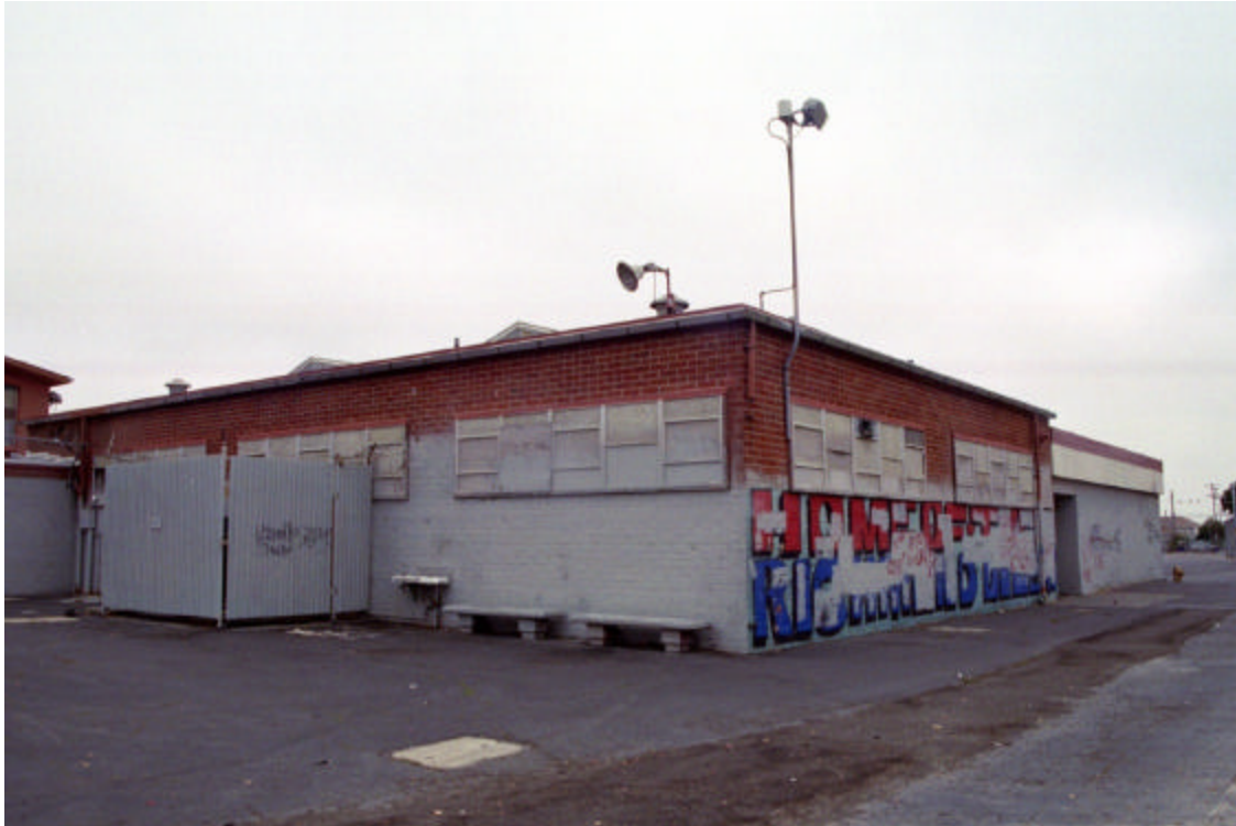
Figure 14: Old Gymnasium Building (Unit B), exterior southeast corner of locker rooms
