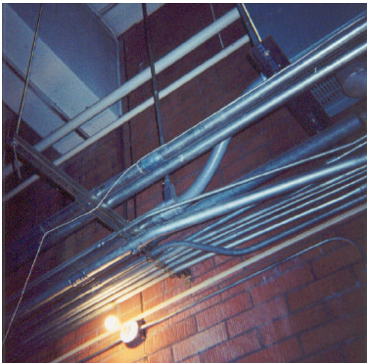
Figure 25: General (Unit D), conduit crossing seismic joint
