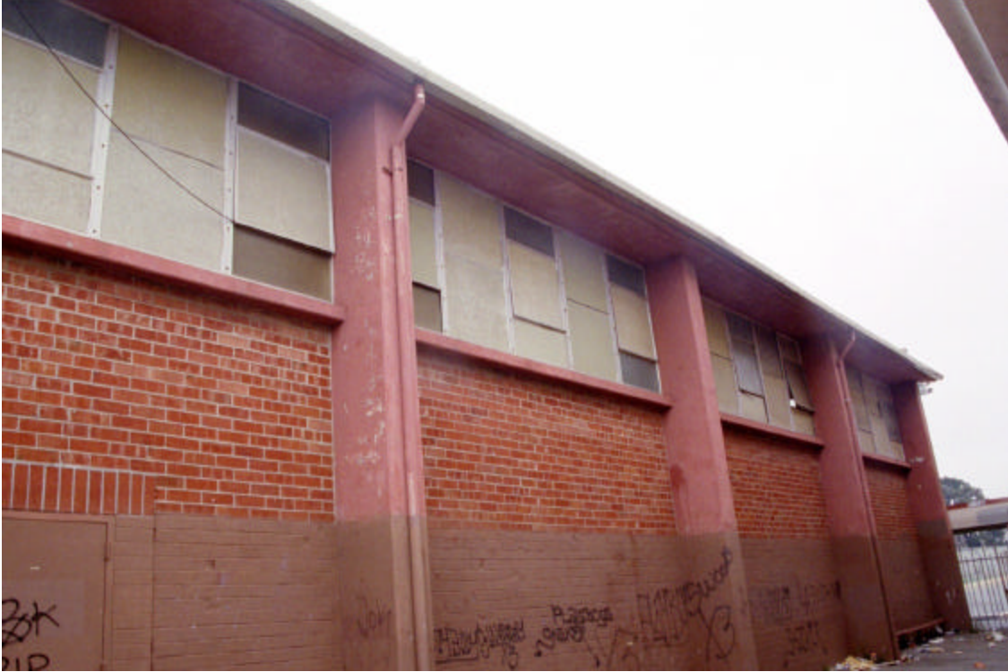
Figure 13: Old Gymnasium Building (Unit B), exterior south wall
