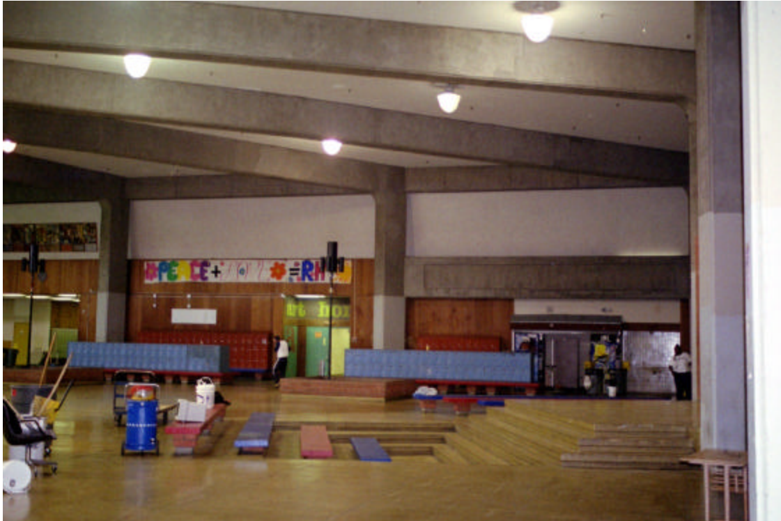
Figure 8: Common Area (Unit D), interior at stage
