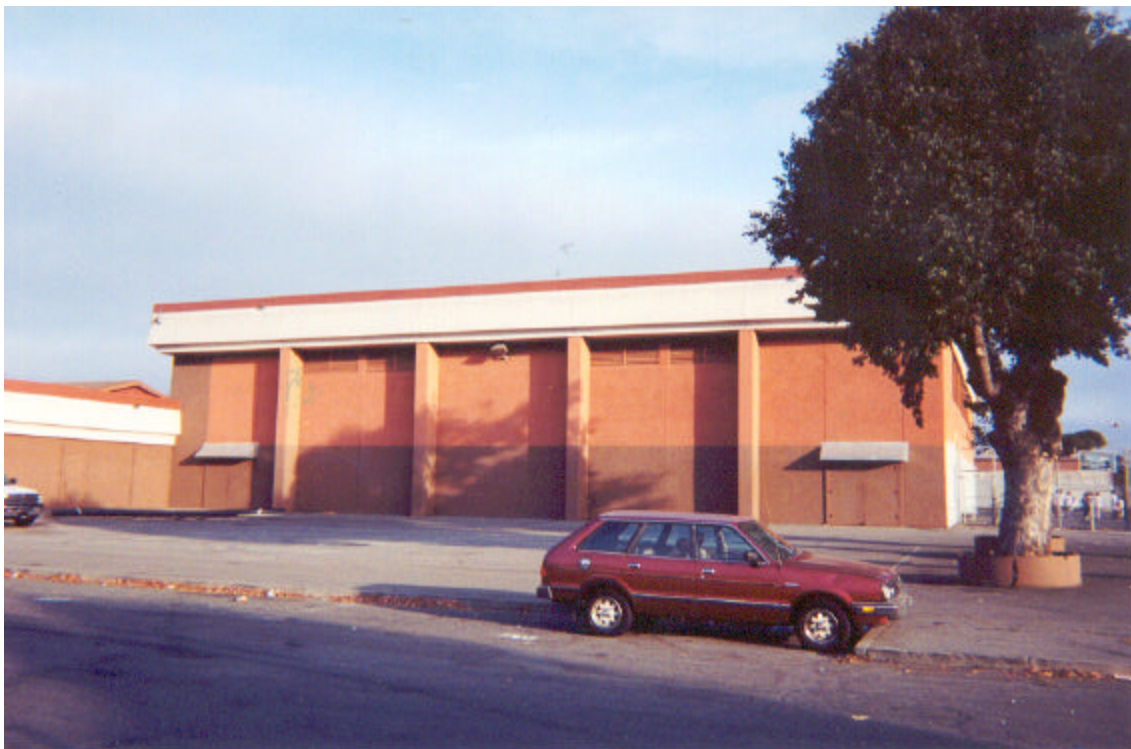
Figure 19: Gymnasium Building (Unit E), exterior south wall
