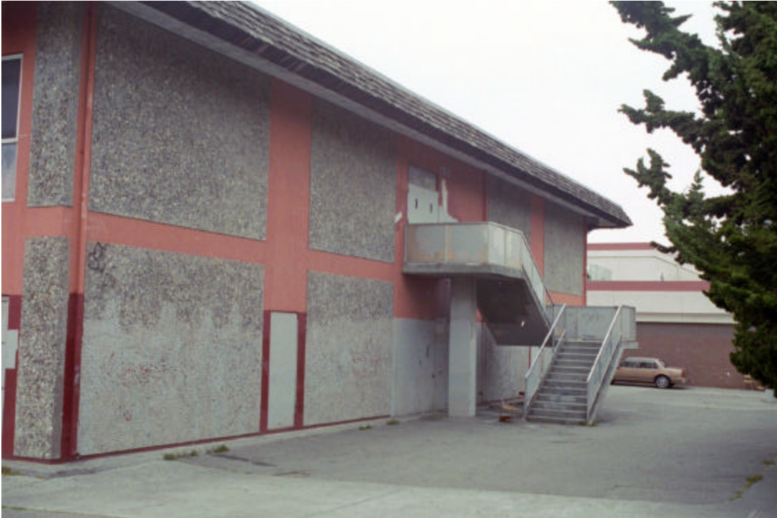
Figure 16: Classroom Building (Unit C), exterior east wall
