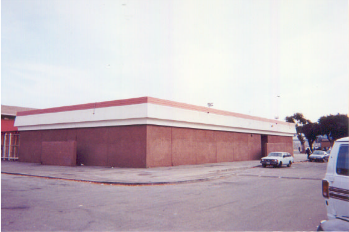
Figure 20: Gymnasium Building (Unit E), exterior southwest corner
