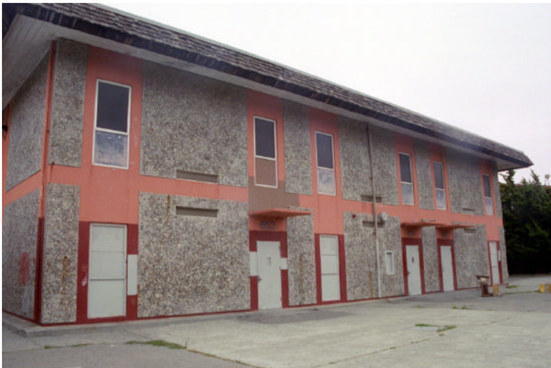
Figure 15: Classroom Building (Unit C), exterior south wall
